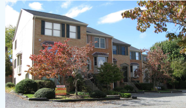
Residential types; townhomes along North Jay Street.
