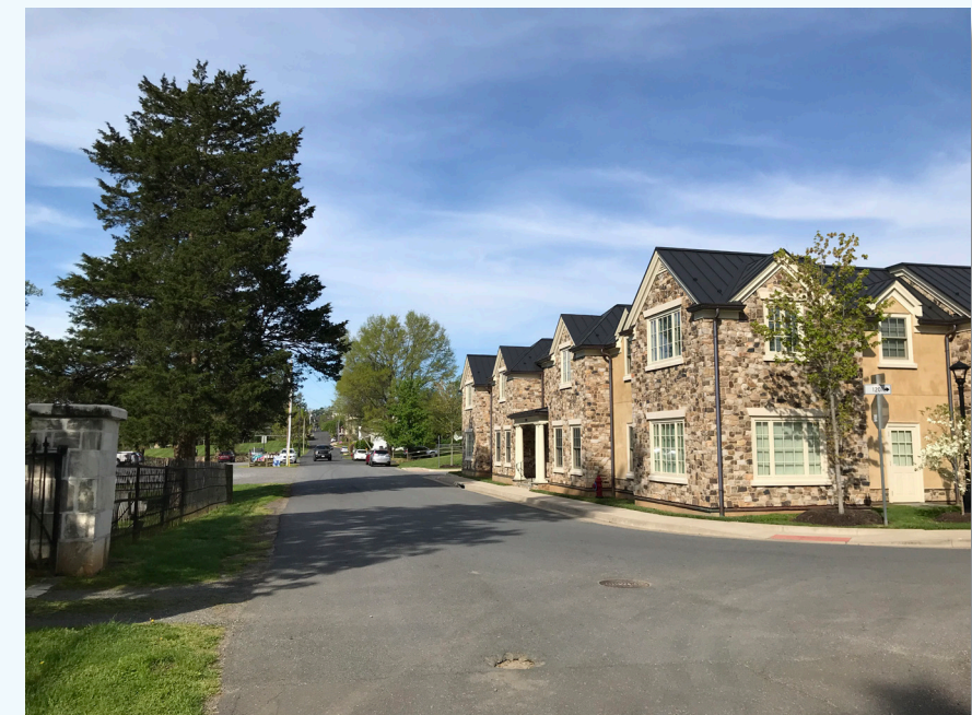
East Federal Street at South Jay Street where new office development has added one small section of curb and sidewalk to the streetscape.
