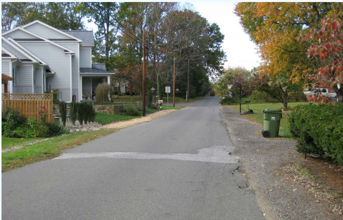
Stonewall Avenue, like many Town streets, is a narrow right-of-way with little traffic and no sidewalk, curb, or pavement markings.
