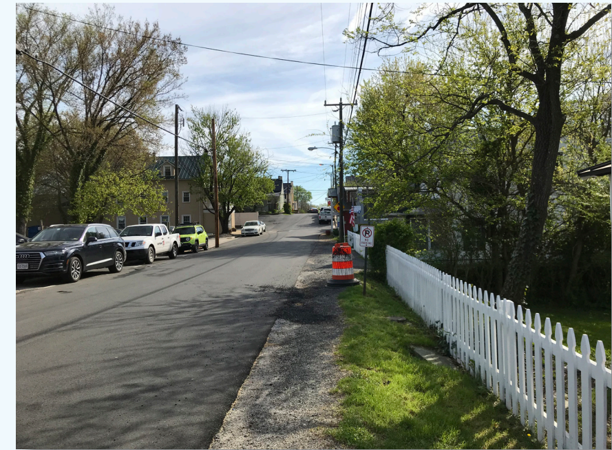
West Federal Street at South Pendleton Street. Much of Federal Street lacks curbs, sidewalks, clearly marked parking, and proper drainage.
