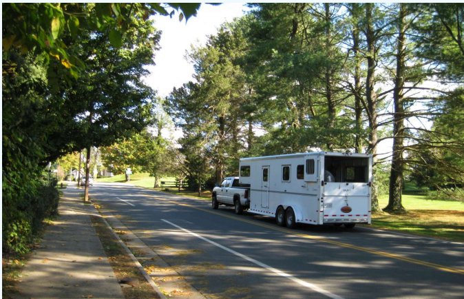
With its wider right-of-way, some areas of Washington Street mix urban (sidewalk & curb) and rural (shoulder & ditch) road design.
