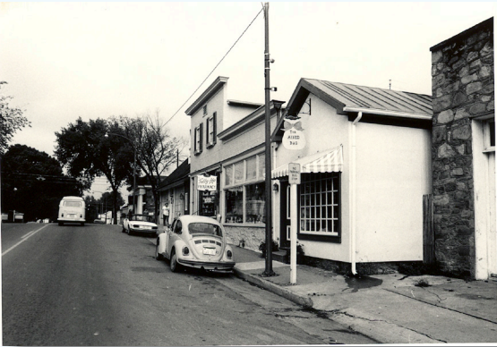
Washington Street before recent streetscape improvements.
